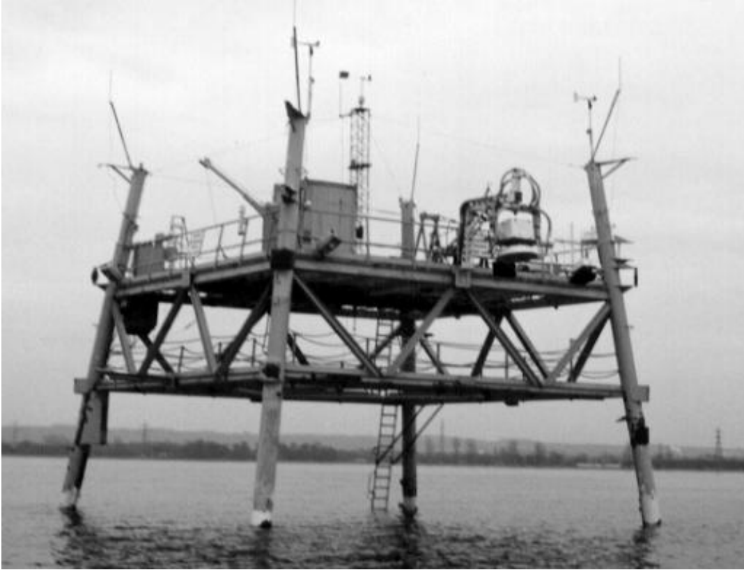
Figure 2.3: The Canada Centre for Inland Waters (CCIW) WAVES research platform. YSCAT is the crane-like structure on the upper deck. Also visible are the two anemometers on the support legs and the bivane anemometer on the tower in the center of the platform.
