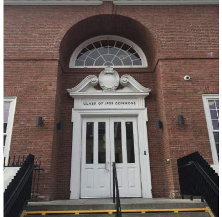
Opening this door requires more effort than opening some other doors.
